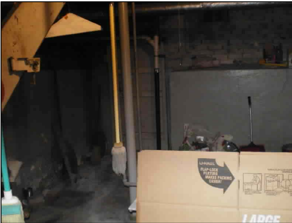
928 Valley Rd Pl GENERAL VIEW 8
