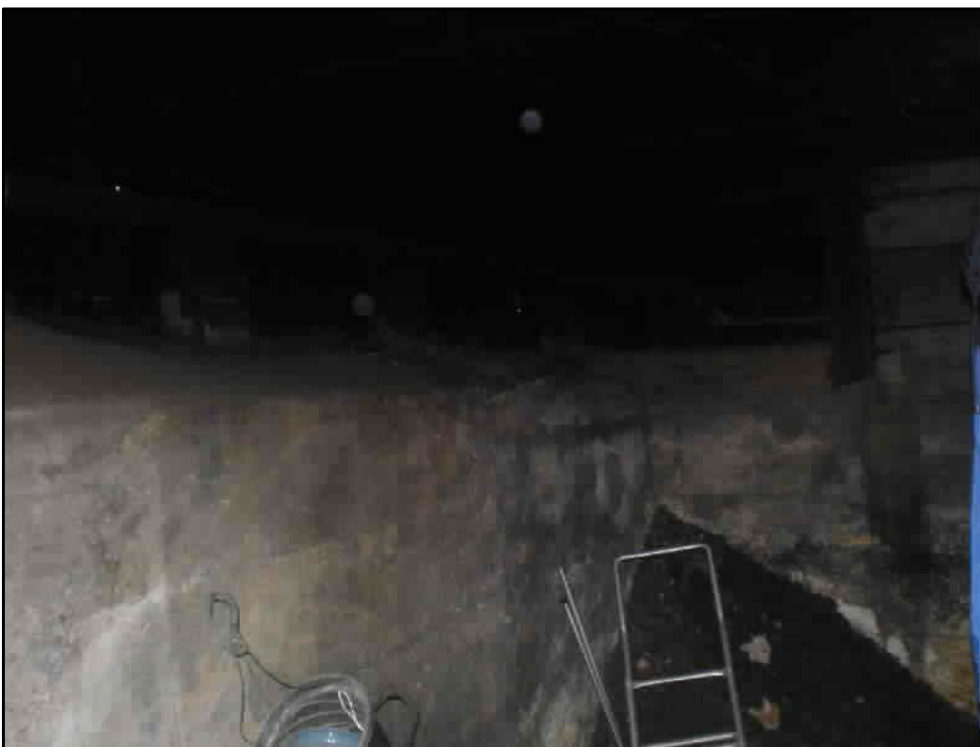
928 Valley Rd Pl GENERAL VIEW 9
