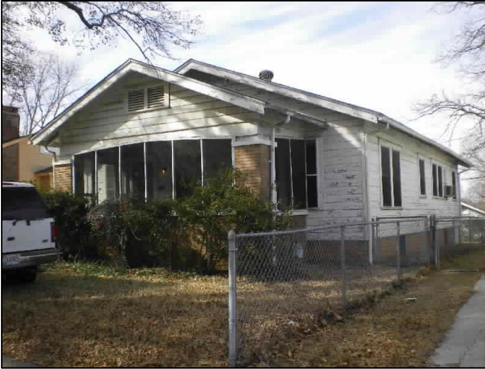
FRONT VIEW OF SUBJECT PROPERTY
