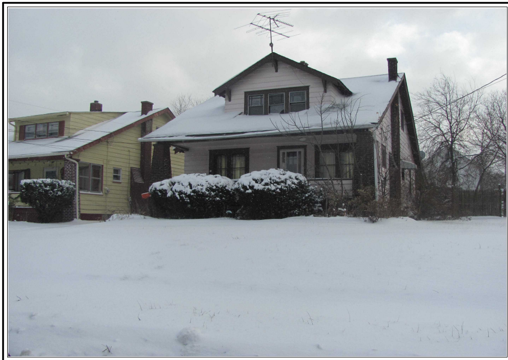
FRONT OF SUBJECT PROPERTY 633 Pasadena Ave. Youngstown, OH 44502
