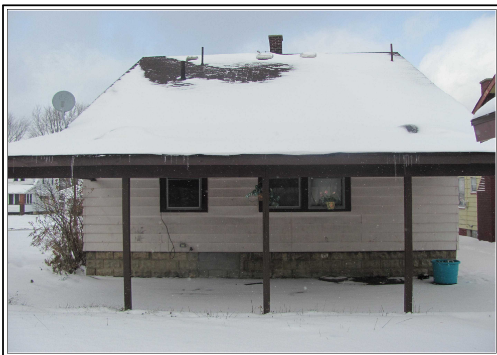
REAR OF SUBJECT PROPERTY
